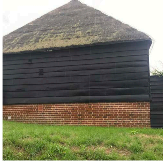
A more ‘rustic’ approach to timber cladding used in Caldecote village. This resonates with the village’s agricultural character.
