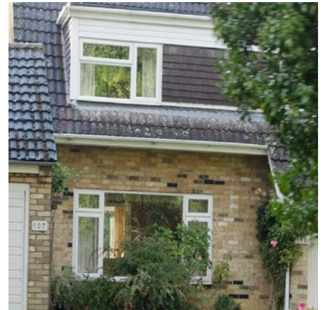
Buff bricks and hung tiles on a chalet dormer on a mid c20 house. Chalet-style windows are commonplace in the village.
