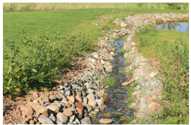
Fig.21 Example of an attractive rural SUDS system within a larger new development. The typical Caldecote ditch is deeper than this example and its banks are greener.
