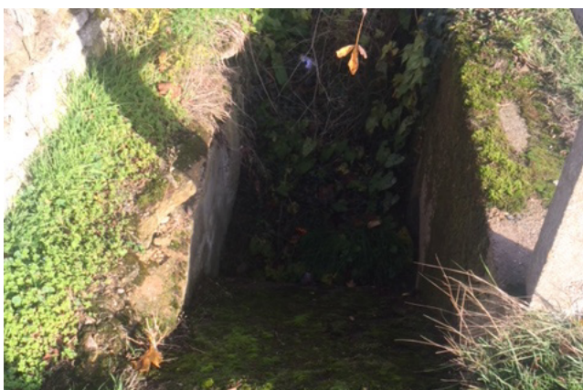
Fig.20 'This represents all the drainage problems of the village. It's a tiny 4" pipe that drains all the surface water from the north of the village. The surface water infrastructure of the village has all been built over. Ditches have been eroded and lost. There were ditches on both sides of the road. Also there's loads of rubbish in there very often.'
