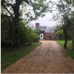
Permeable vehicle access lined with grass
